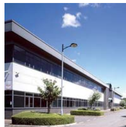
Redhill Data Centre. Redhill. Great Britain.
